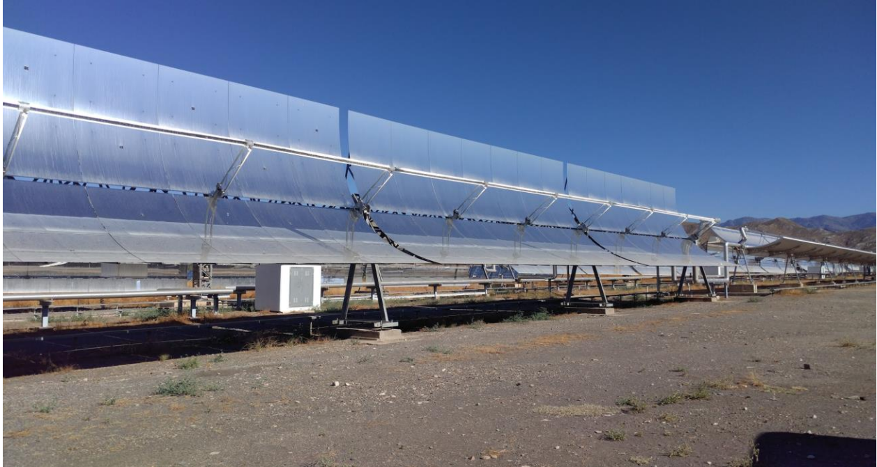
Image 11: Thermosolar power plant with parabolic cylinders
