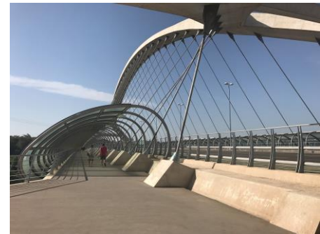
Image 13: A newly constructed bridge in Spain
